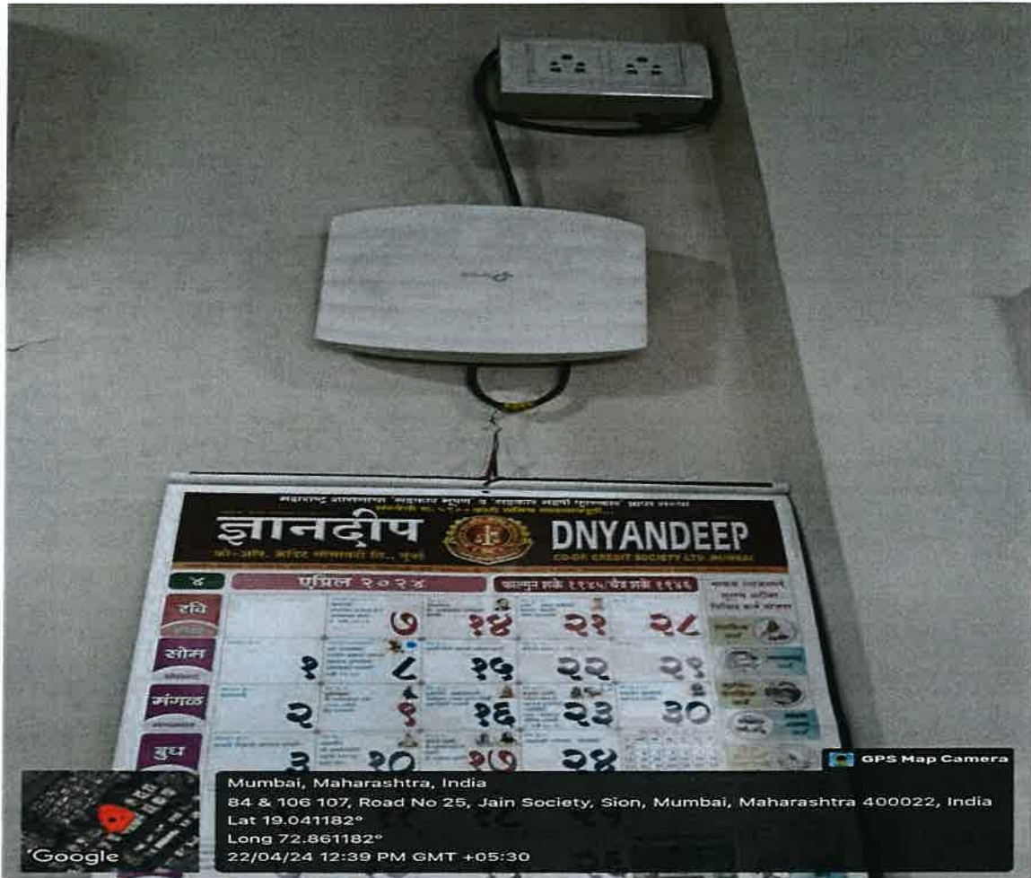
Academic Staff Centre installed since 2018-19.
